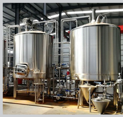
Milk Processing Plant
